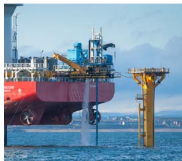
Figure 4: The MPI Adventurer installing the anemometry hub off Blyth. Courtesy of Steve McDonald
